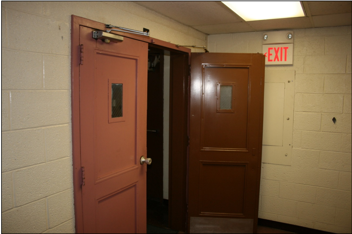
Figure 47: Building 3-1, interior door detail
