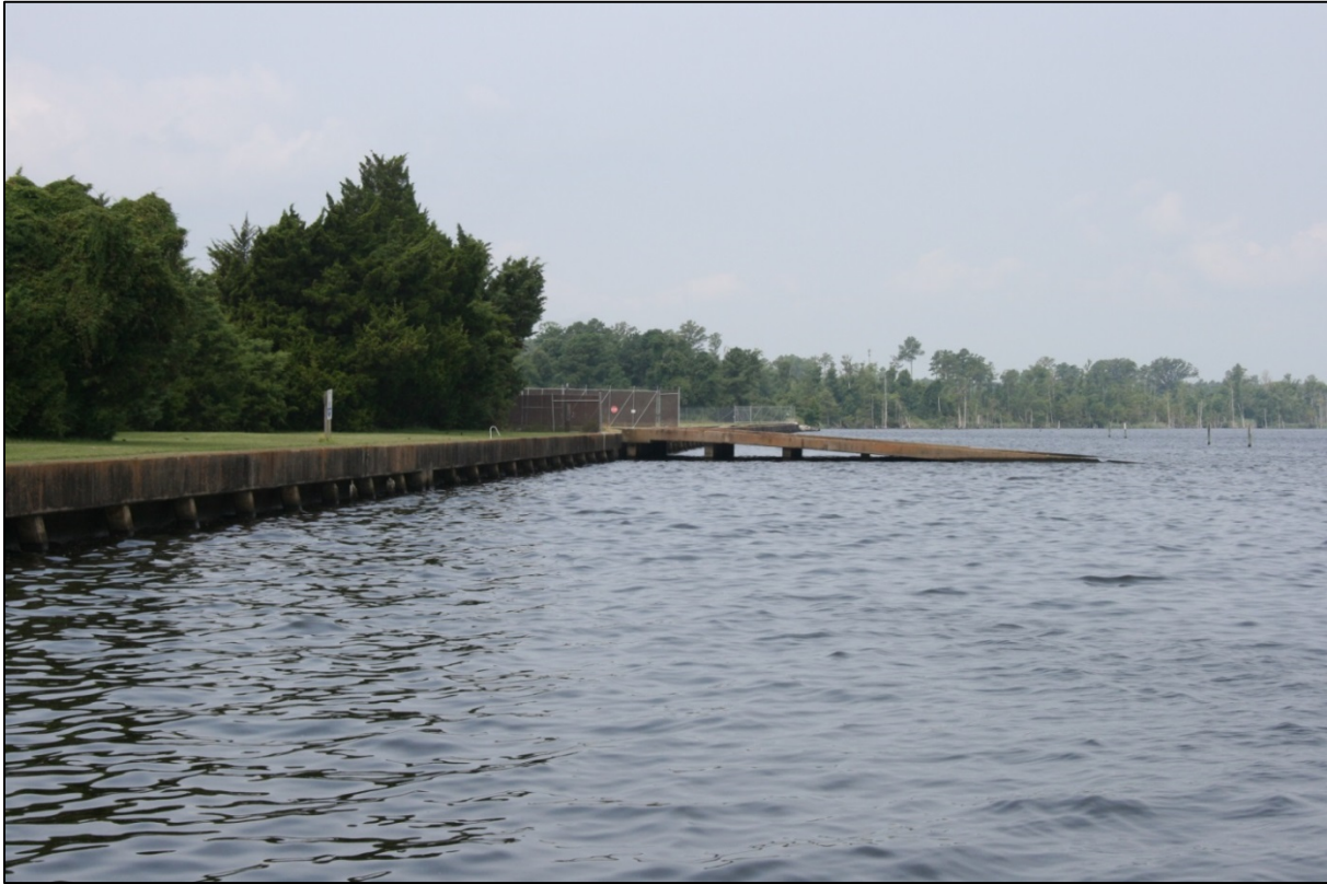
Figure 66: Facility 3-11 looking west
