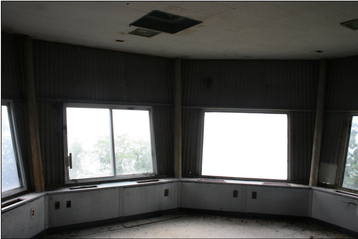
Figure 38: Building 1-14, control room detail view looking east
