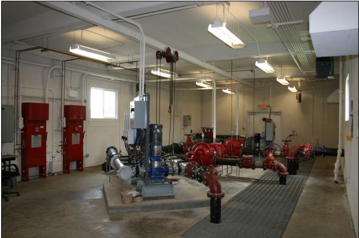
Figure 90: Building 5-6, interior view, looking southwest
