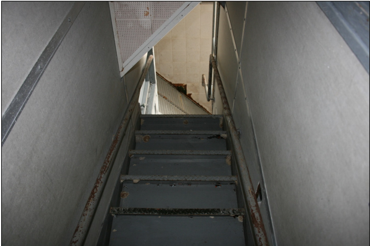
Figure 35: Building 1-14, interior stair detail
