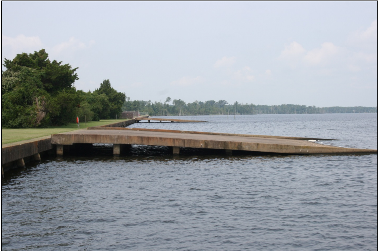
Figure 65: Facility 3-10, in foreground, Facility 3-11, in background looking west
