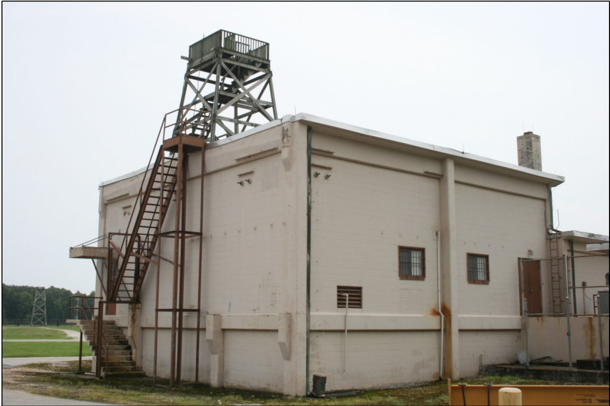
Figure 2: Building 6-1, north and east elevations
