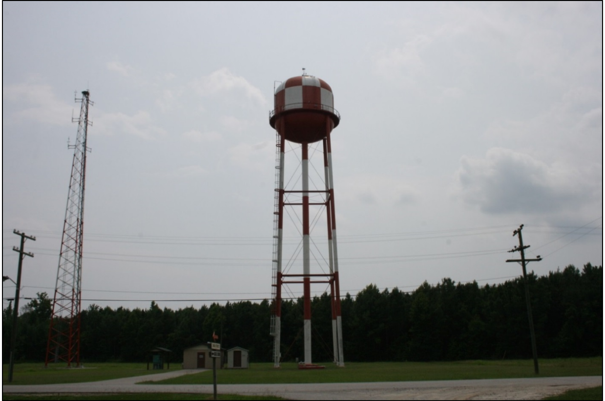
Figure 108: Building 8-4 looking south
