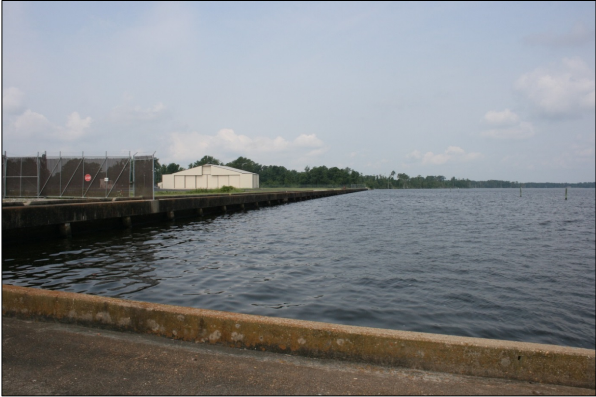
Figure 67: Facility 3-11, view from the ramp to the shoreline looking south
