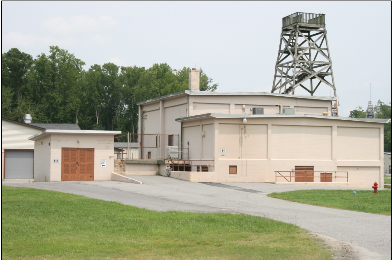
Figure 98: Building 6-1, south (front) and west elevations
