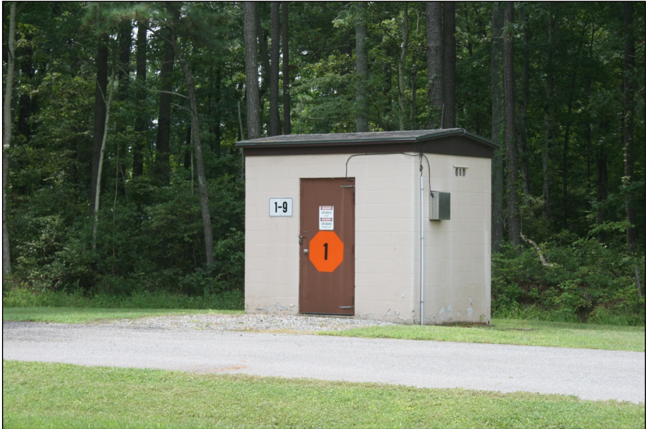
Figure 28: Building 1-9, north and east elevations
