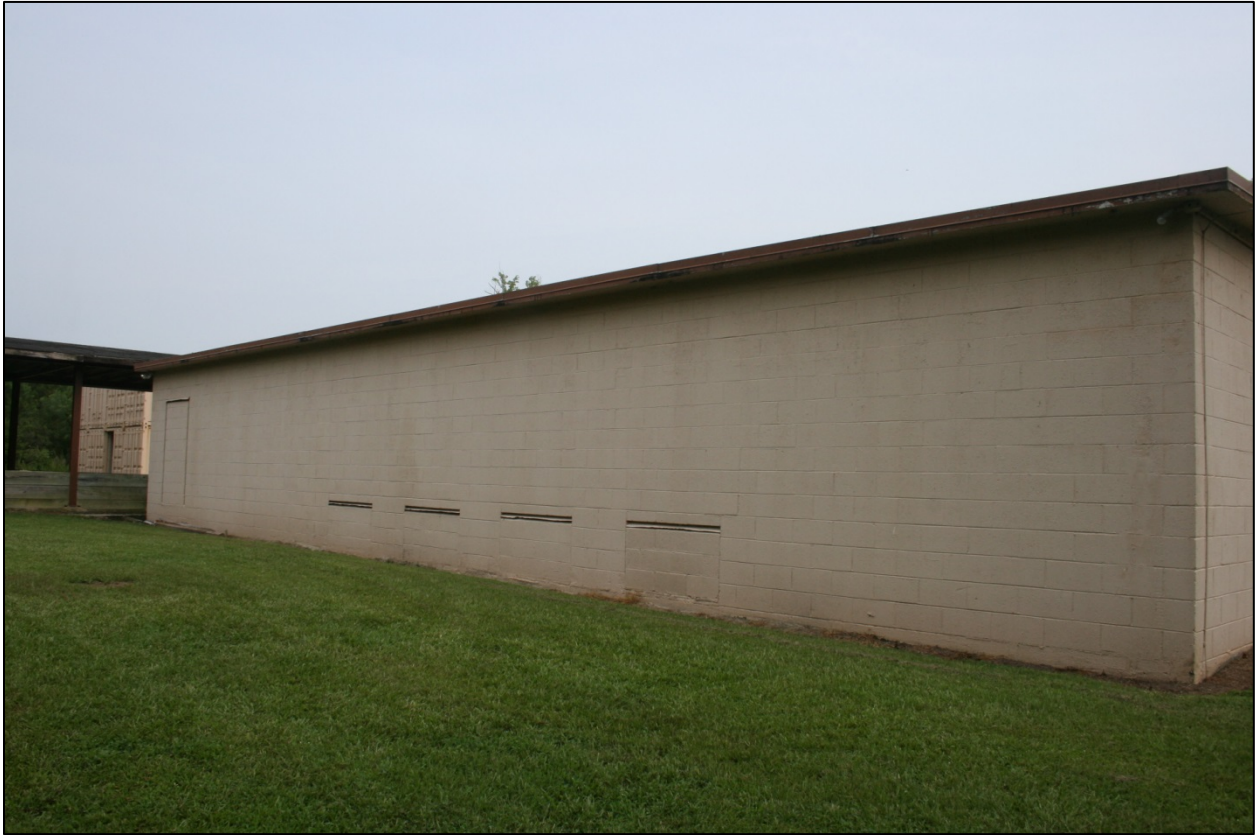
Figure 31: Building 1-13, rear (south) elevation
