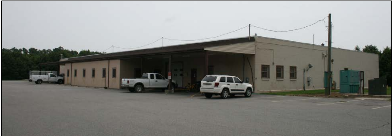
Figure 85: Building 5-2, north and west elevations
