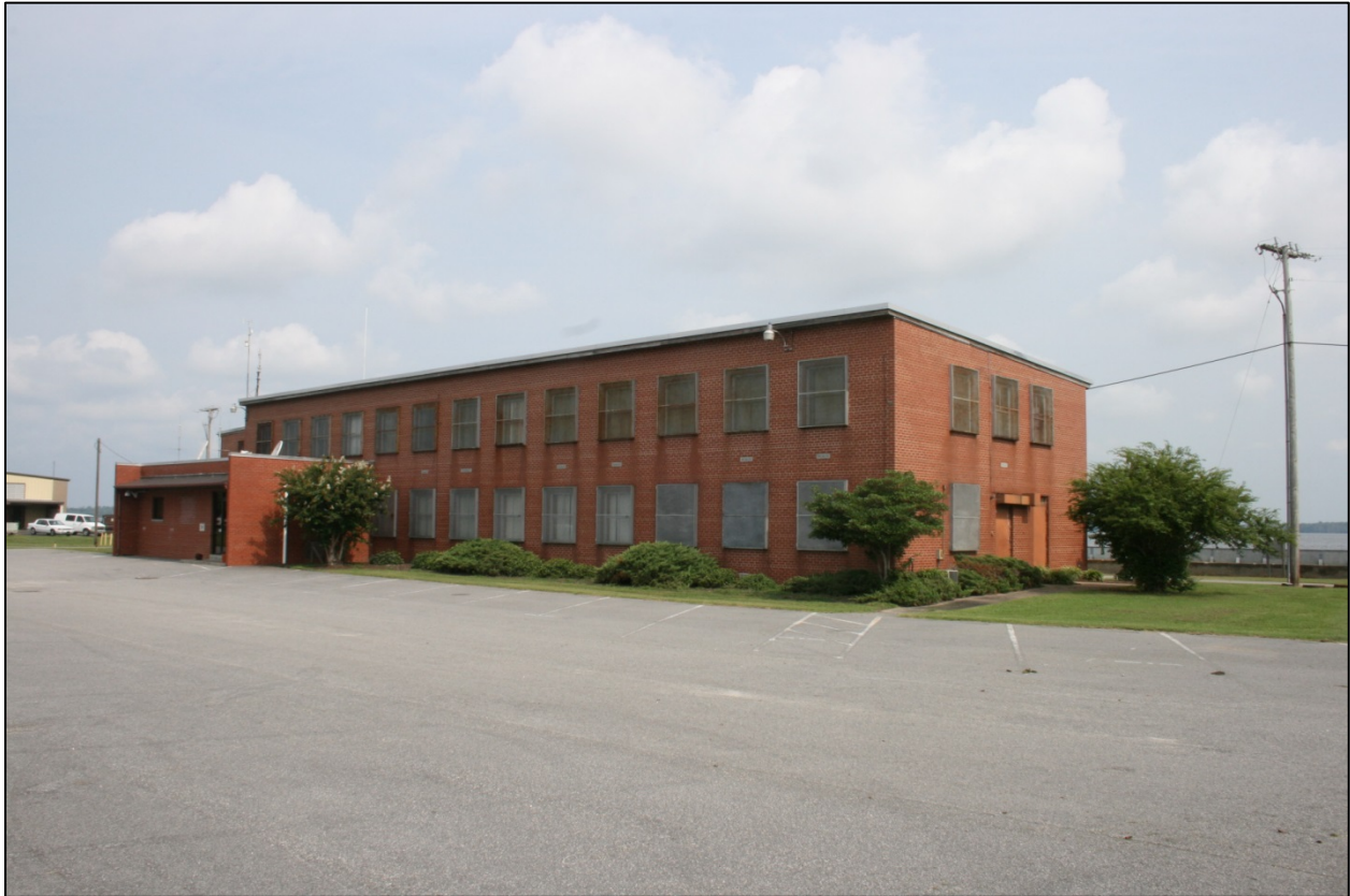
Figure 39: Building 3-1, front (south) and east elevations
