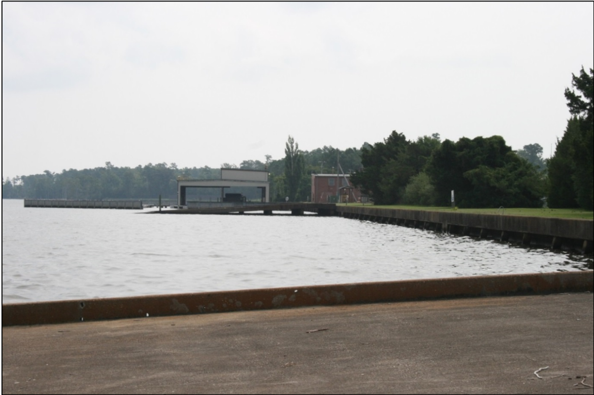
Figure 68: From Facility 3-11 with a view to Facility 3-10 looking east
