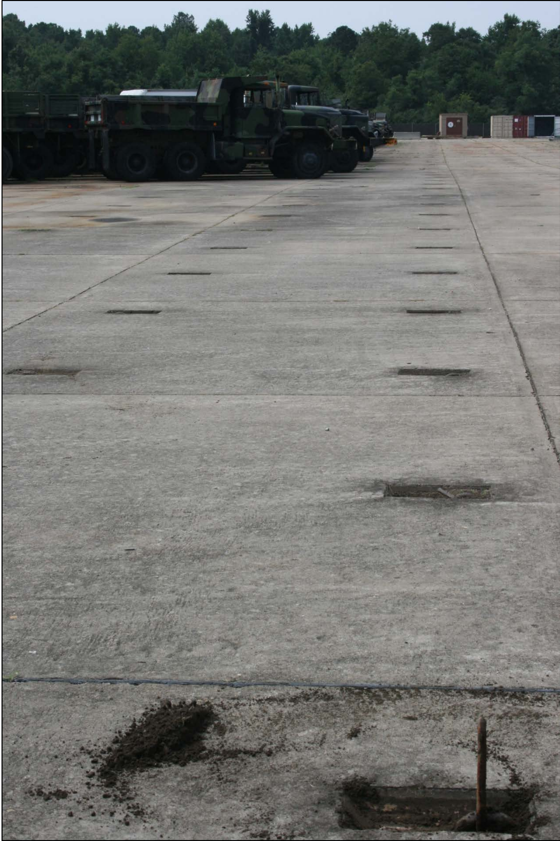
Figure 76: Facility 3-12, general view showing apron hooks
