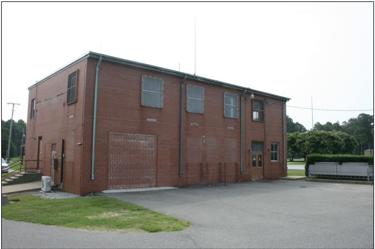
Figure 44: Building 3-1, north and west elevations
