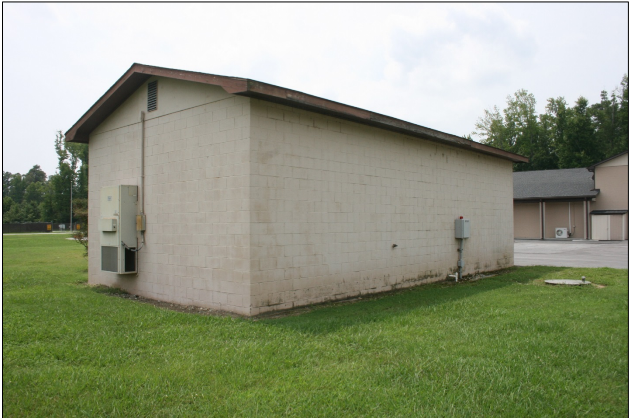
Figure 105: Building 6-4, north and east elevations
