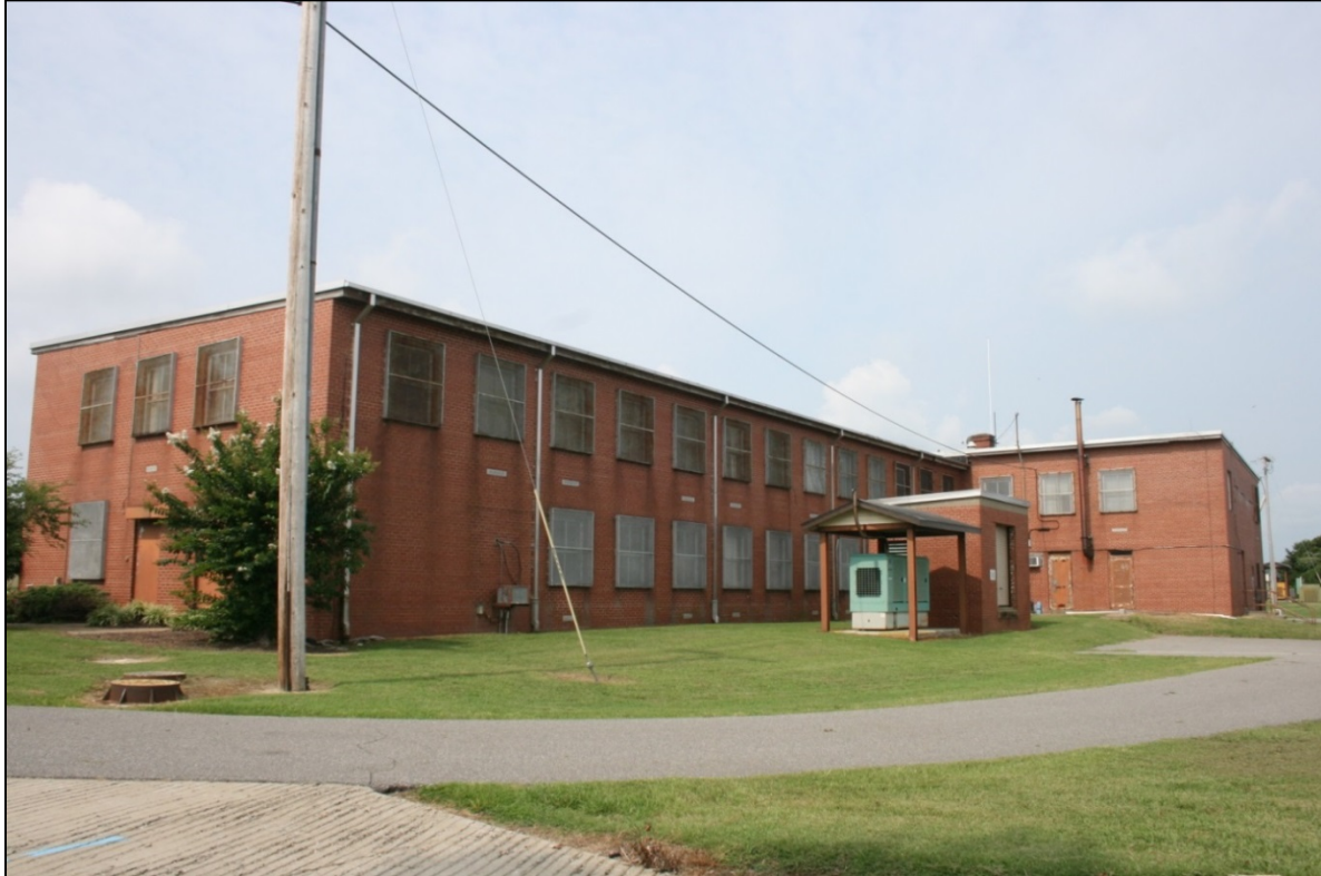
Figure 43: Building 3-1, north (rear) and east elevations
