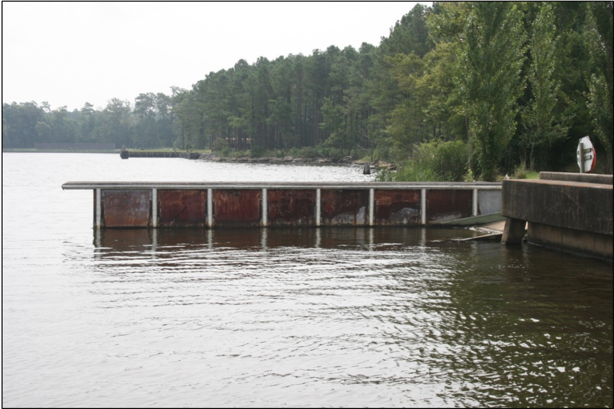
Figure 58: Building 3-2, view of associated breakwater
