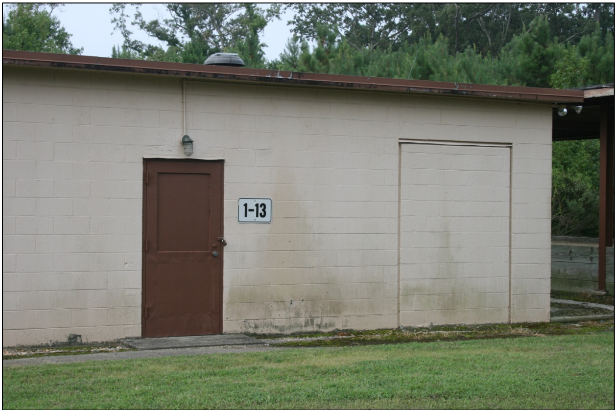
Figure 30: Building 1-13, front (north) elevation, detail
