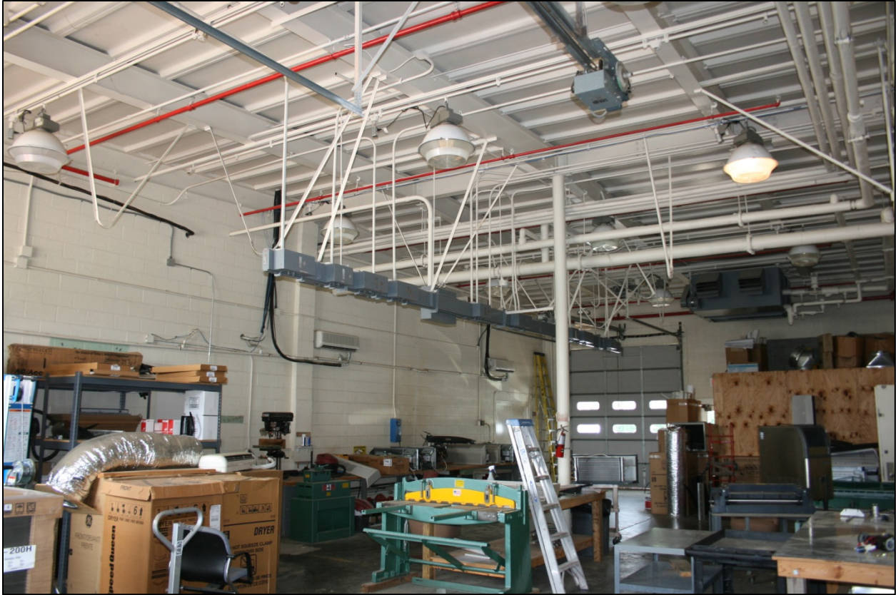
Figure 82: Building 5-1, interior workshop area (east portion of the building)
