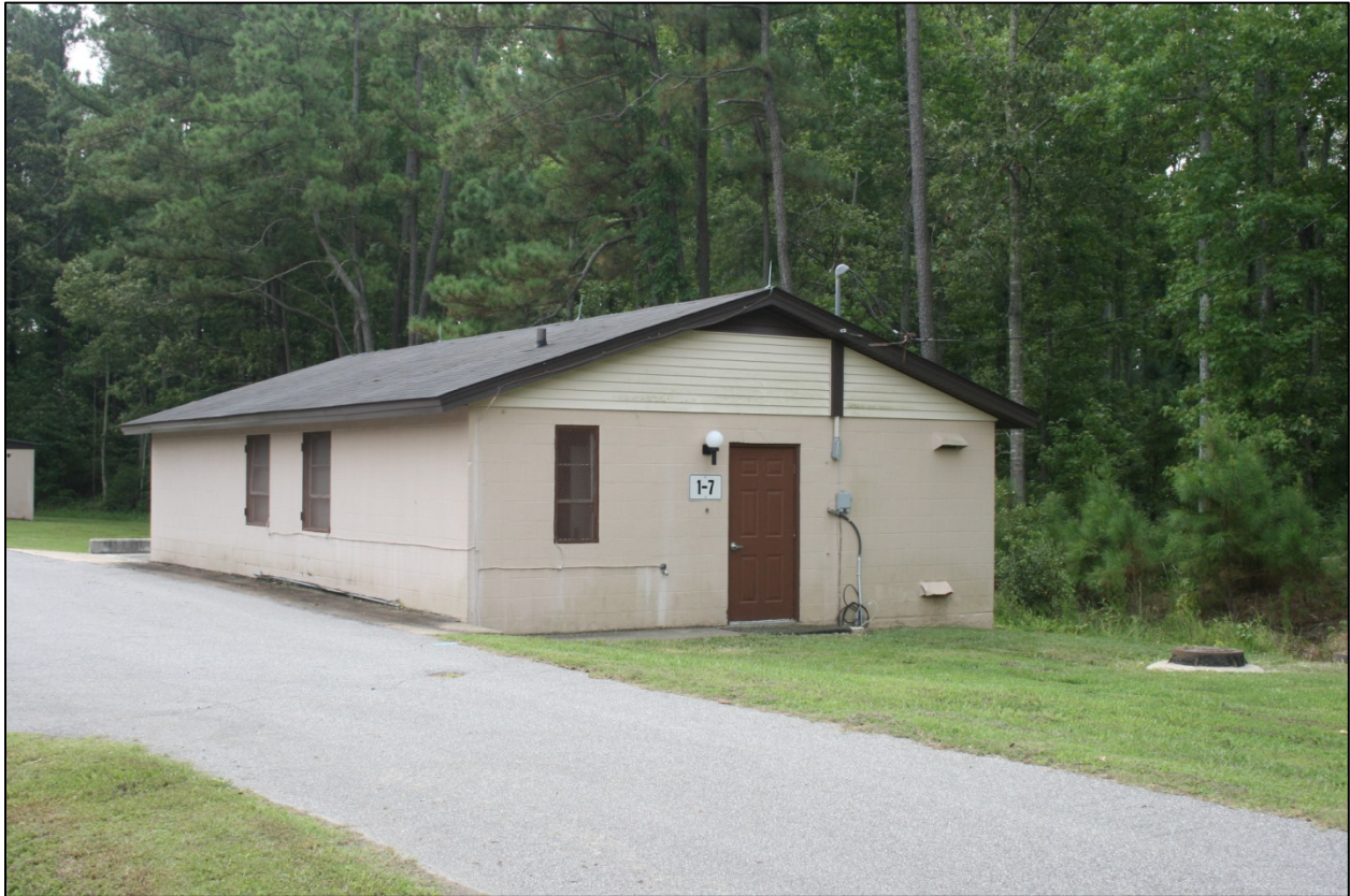
Figure 26: Building 1-7, north and east elevations
