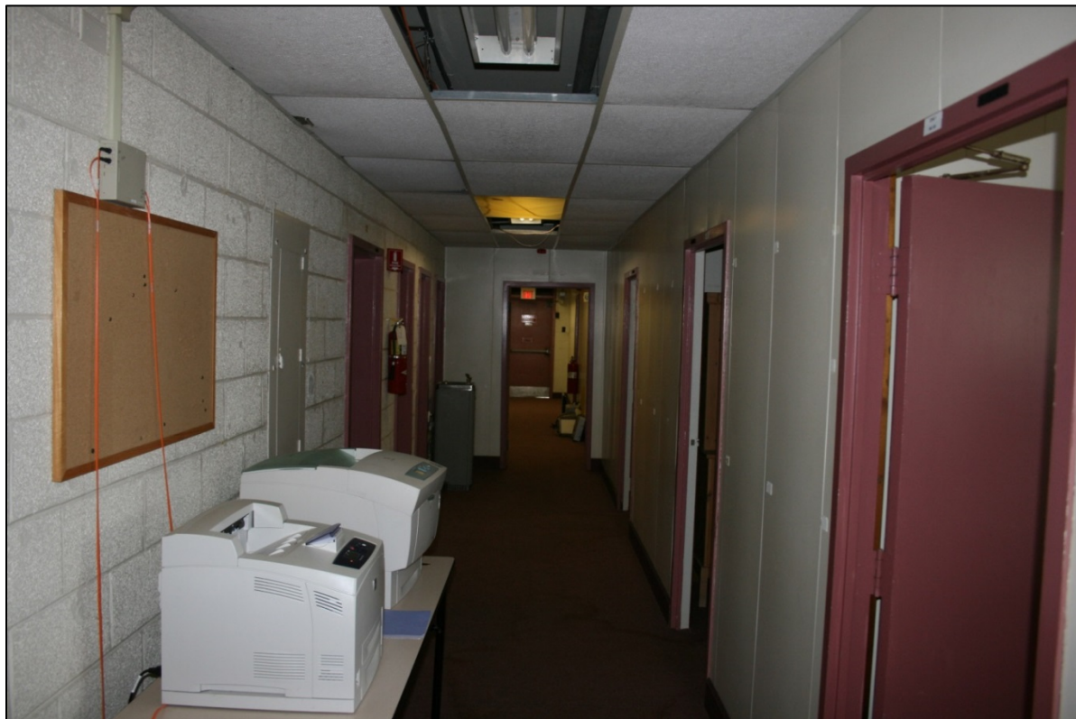
Figure 46: Building 3-1, interior hallway
