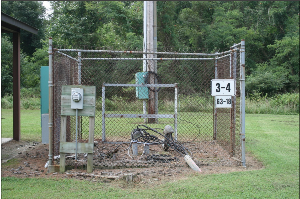
Figure 64: Building 3-4 looking south
