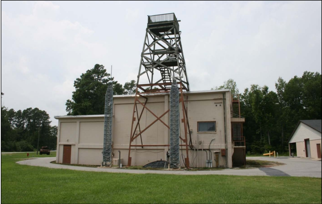
Figure 100: Building 6-1, east elevation
