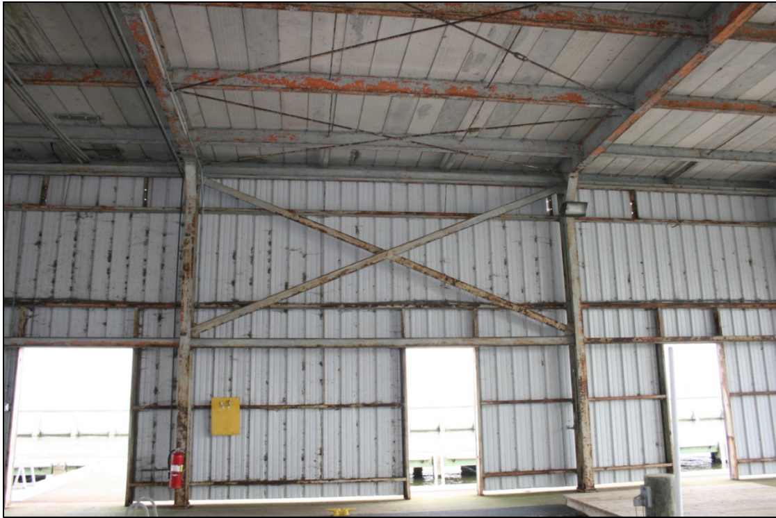
Figure 59: Building 3-2, interior framing detail
