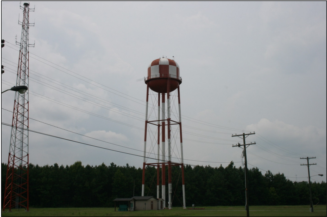
Figure 107: Building 8-4, looking west
