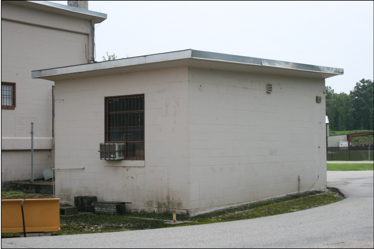
Figure 103: Building 6-2, north and west elevations
