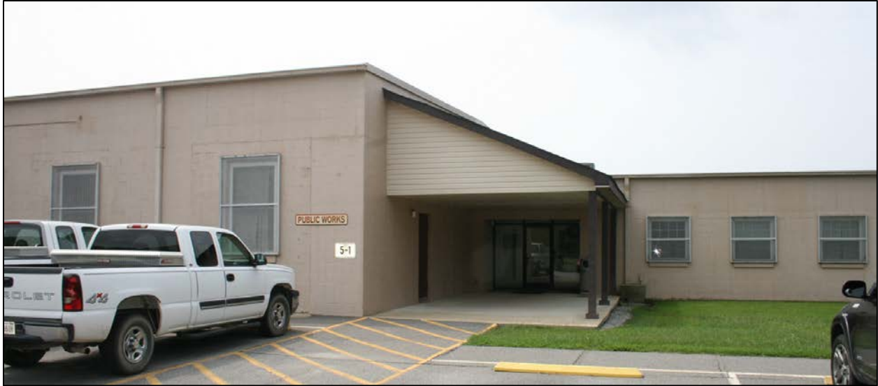
Figure 79: Building 5-1, front (north) entrance detail
