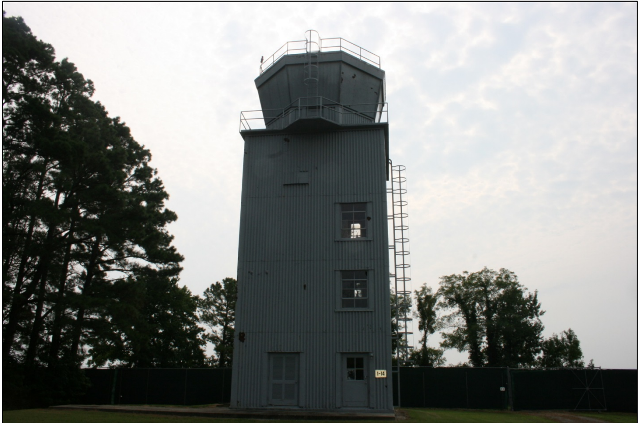
Figure 32: Building 1-14, west elevation
