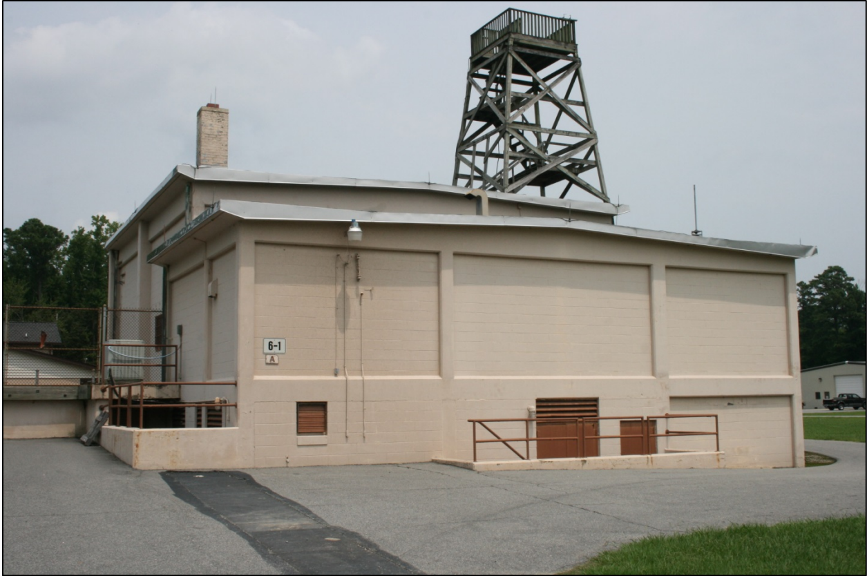
Figure 99: Building 6-1, south elevation
