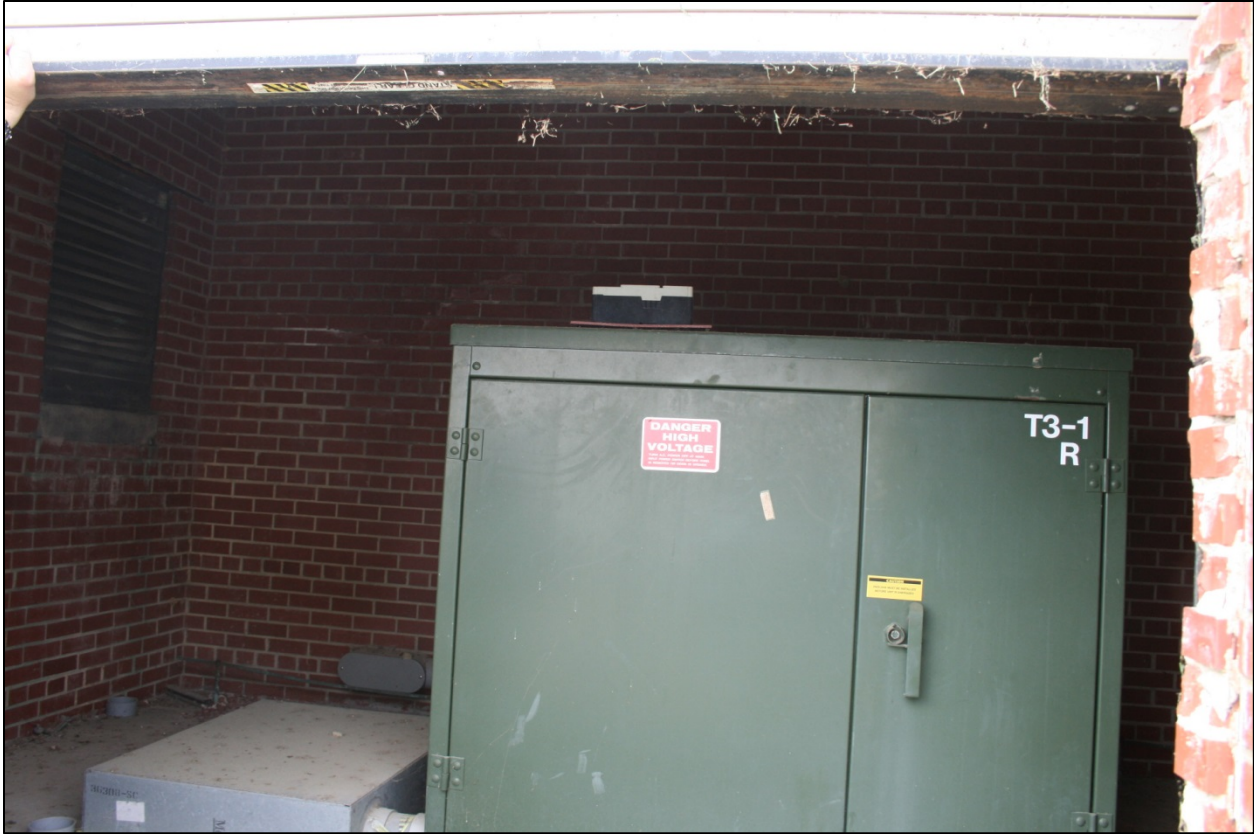
Figure 63: Building 3-3, interior view looking south
