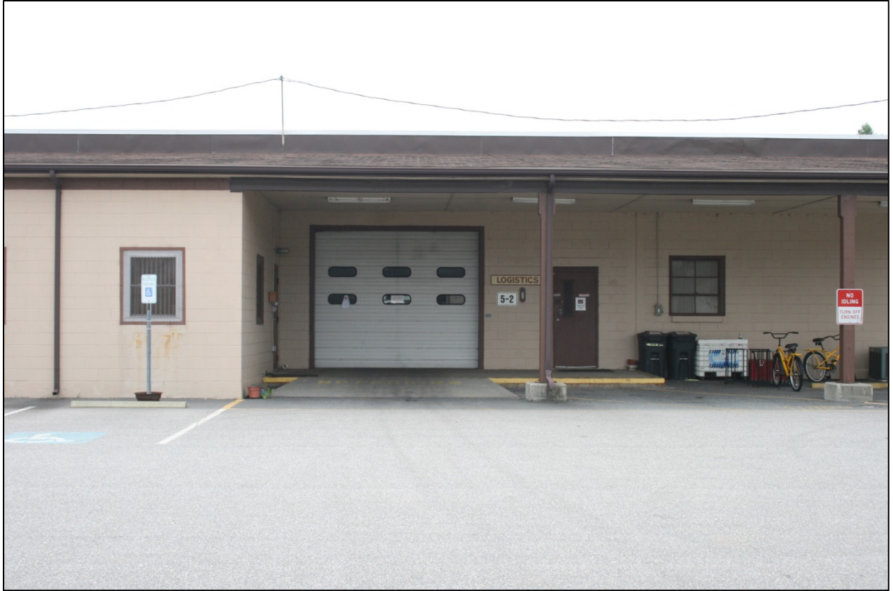
Figure 86: Building 5-2, front entrance and loading area detail
