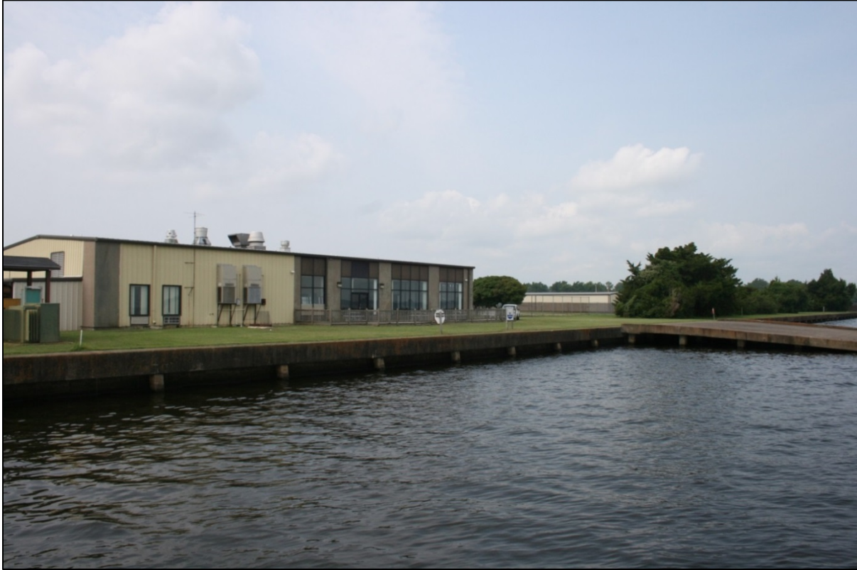
Figure 70: Facility 3-10 looking southwest
