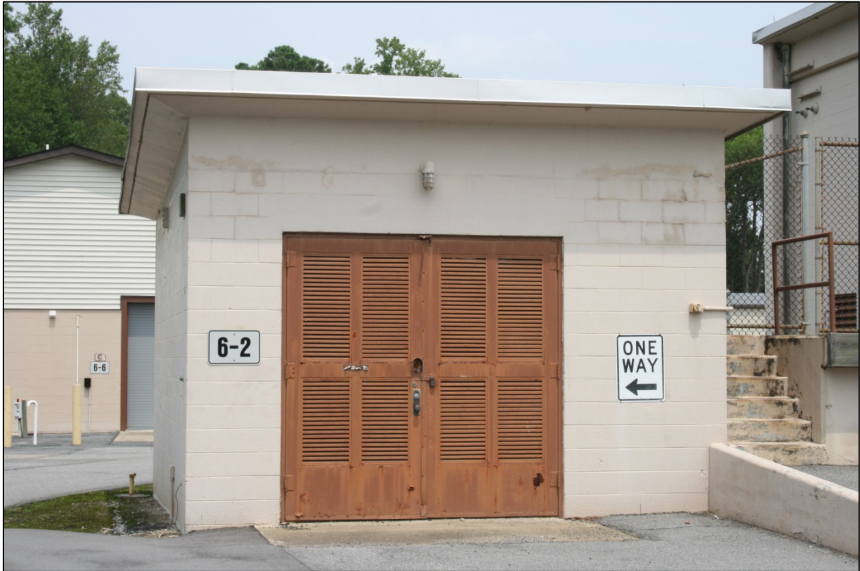
Figure 102: Building 6-2, front (south) elevation
