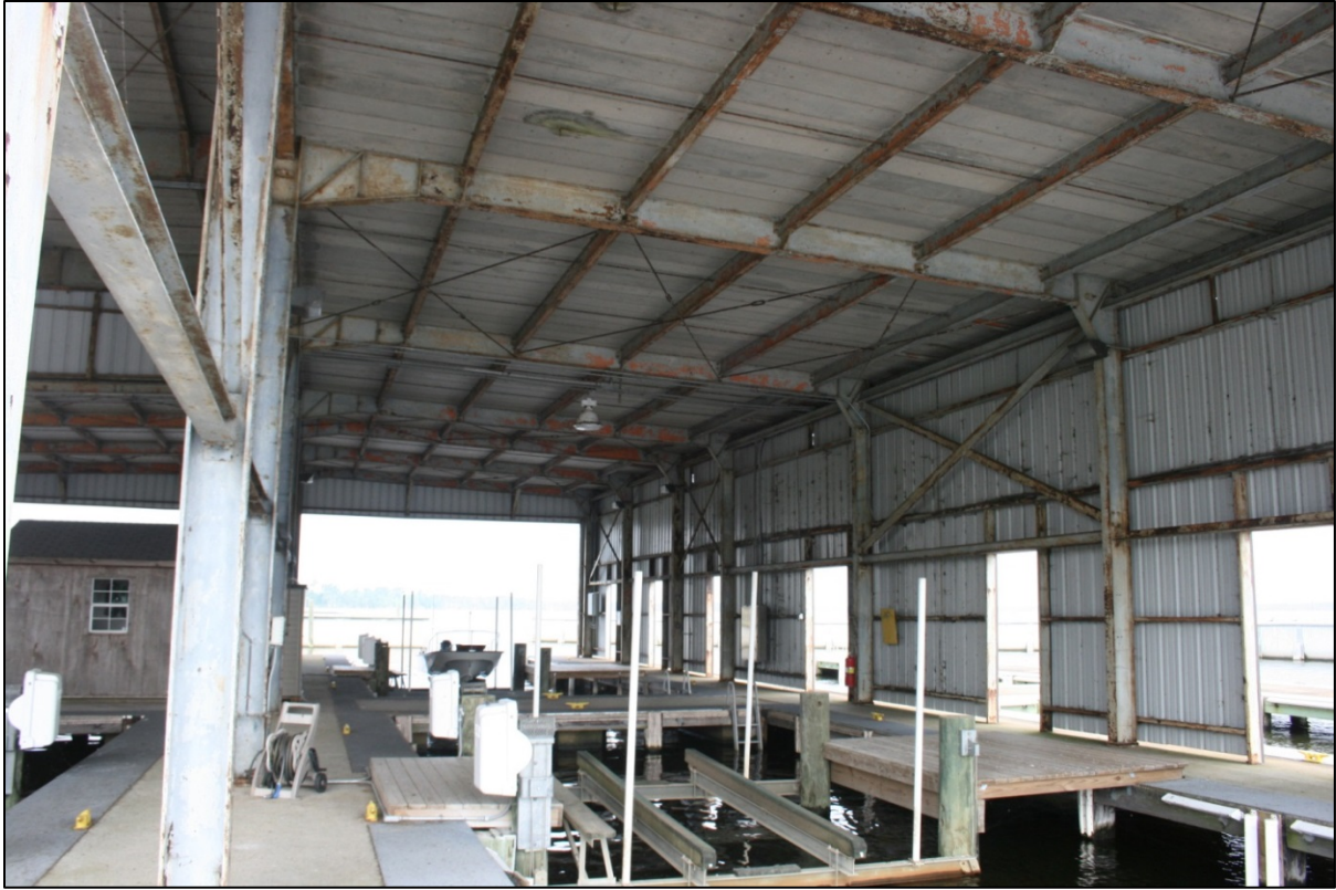
Figure 57: Building 3-2, interior view
