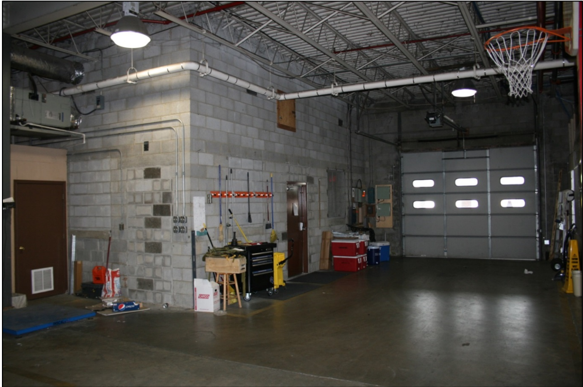
Figure 88: Building 5-2, interior view of office and loading door
