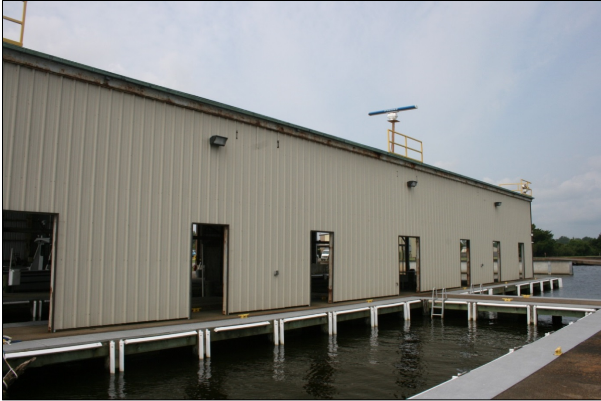
Figure 54: Building 3-2, exterior view of north elevation and docks
