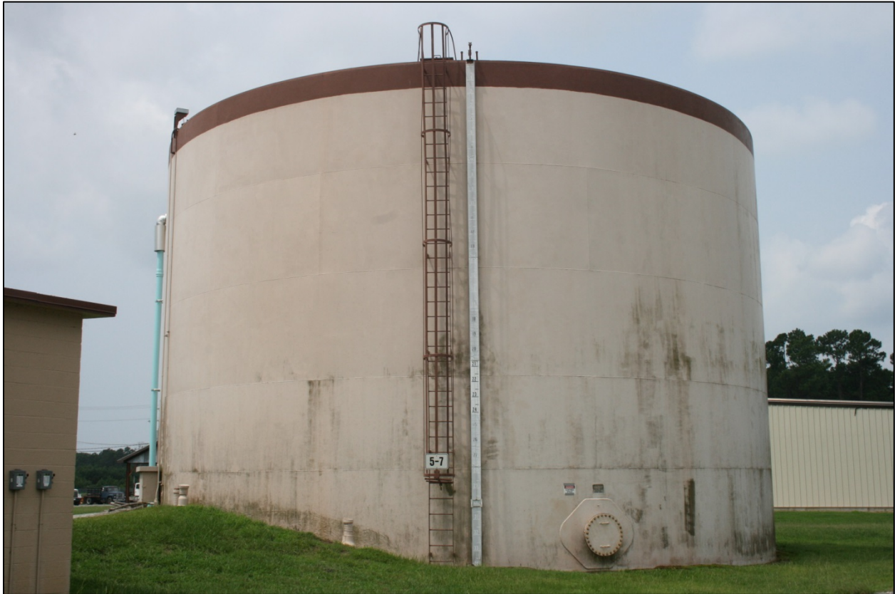
Figure 91: Facility 5-7, looking southwest
