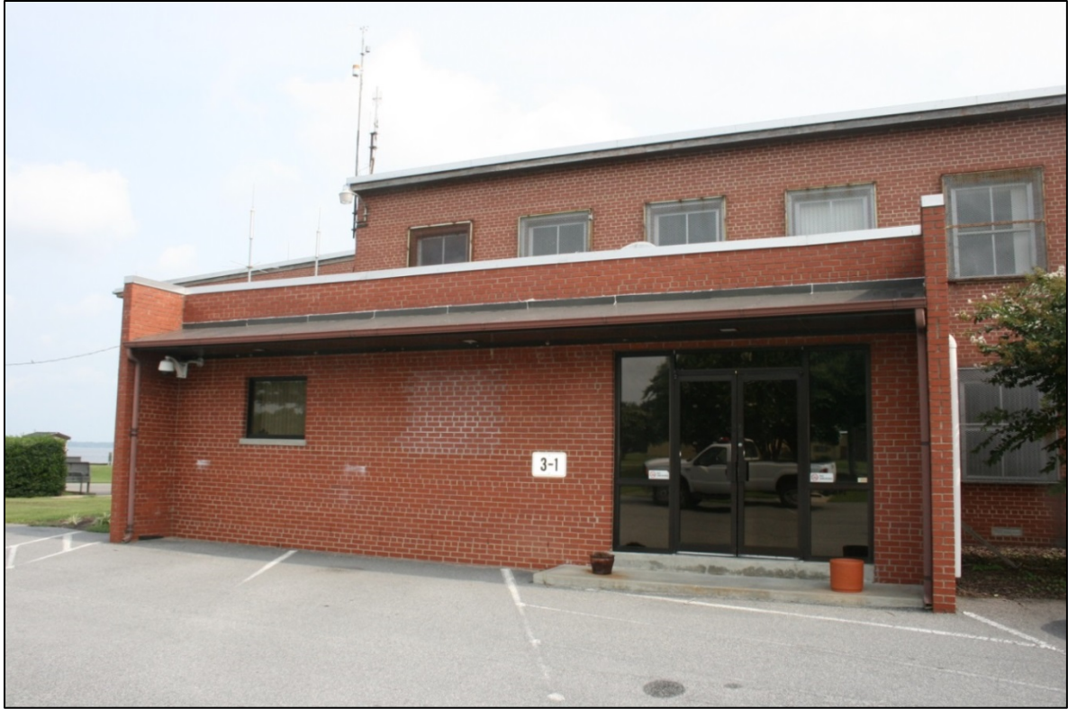
Figure 42: Building 3-1, front entrance detail
