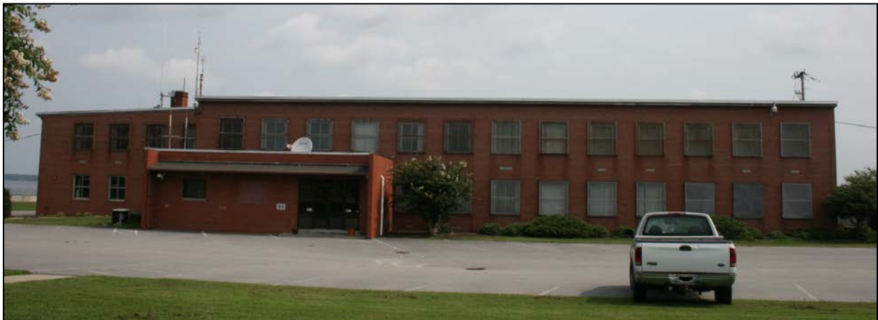
Figure 40: Building 3-1, front (south) elevation
