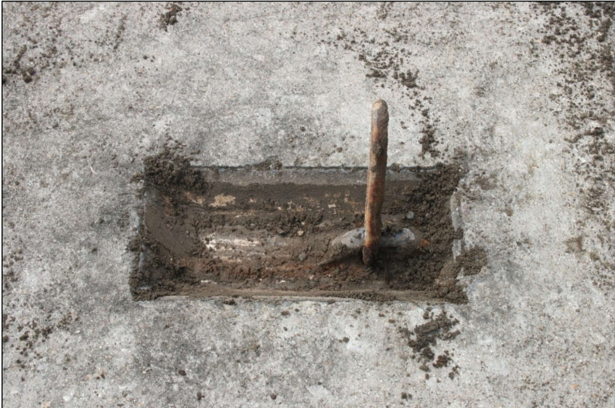
Figure 75: Facility 3-12, apron hook detail
