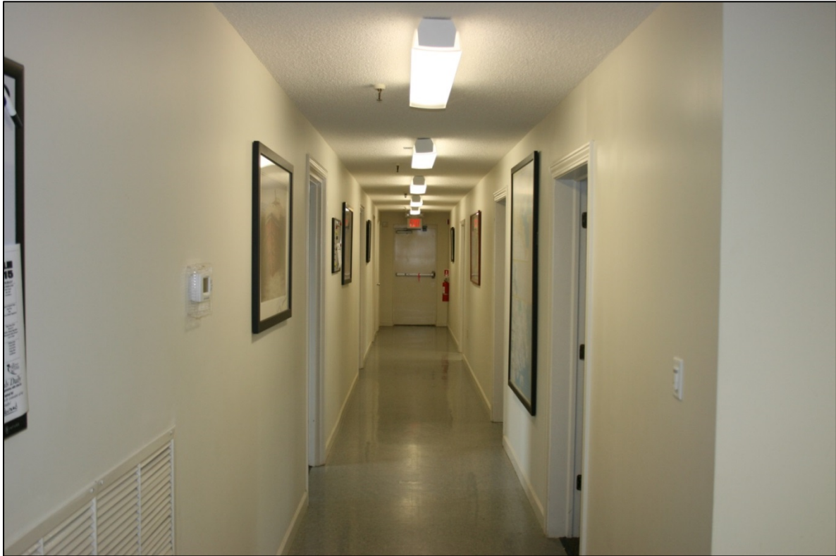
Figure 84: Building 5-1, interior hallway
