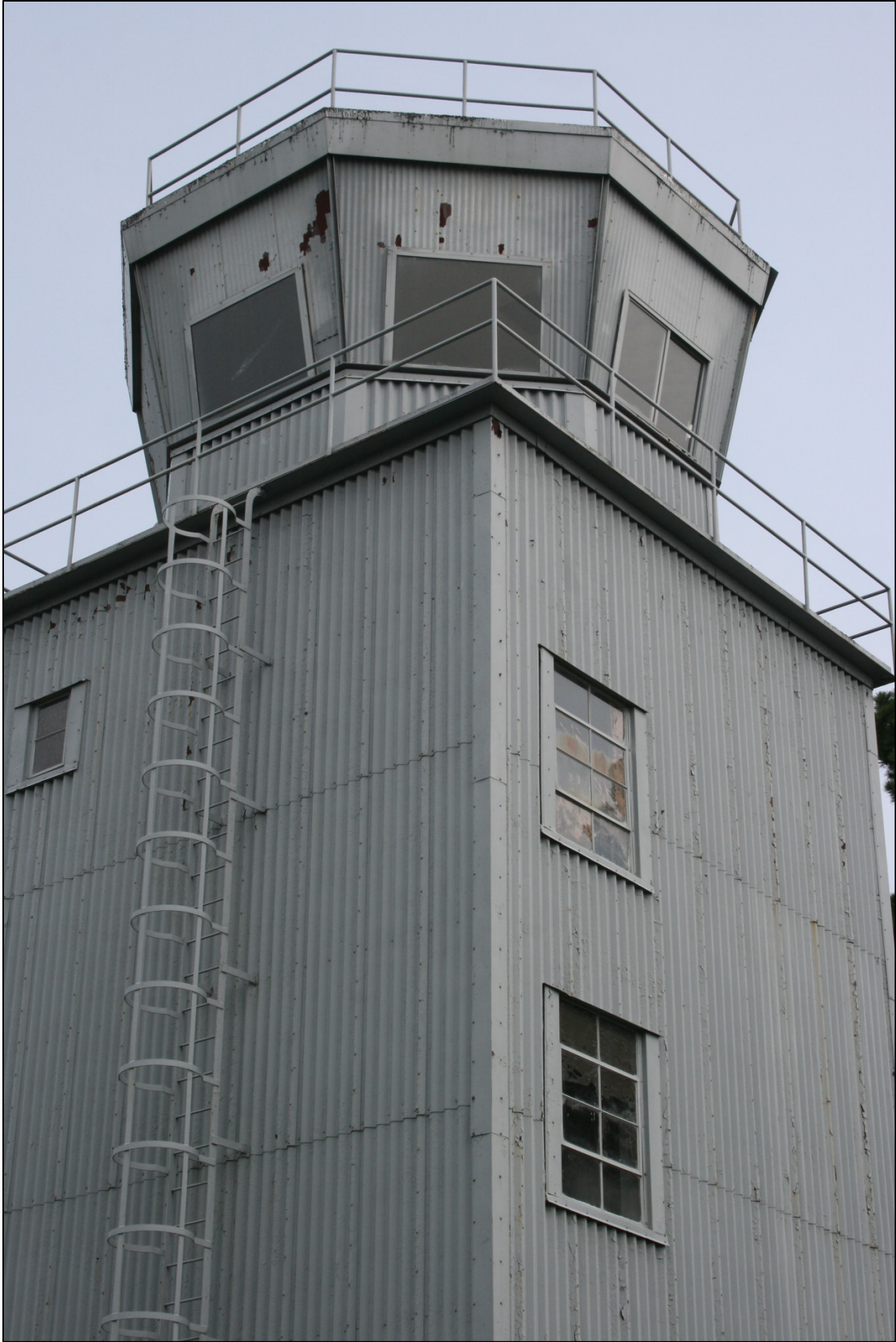
Figure 34: Building 1-14, exterior top floor detail
