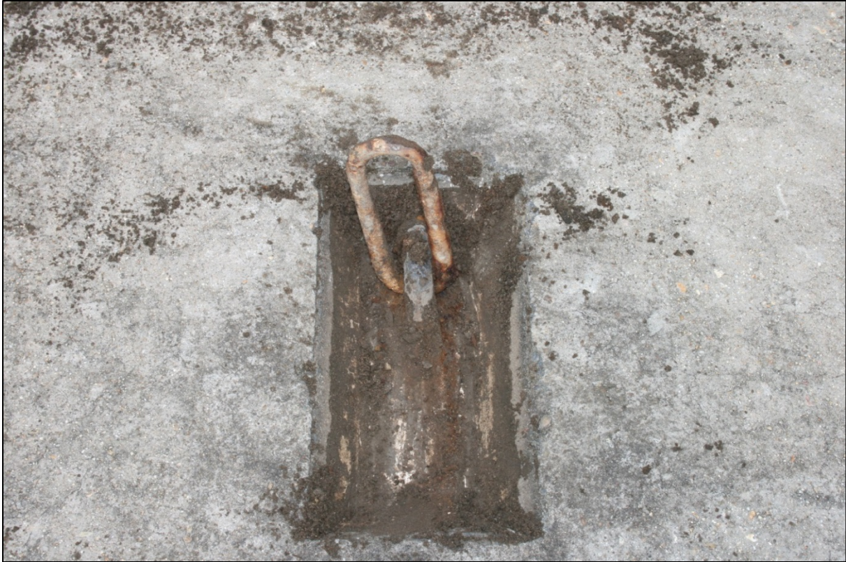
Figure 74: Facility 3-12, apron hook detail
