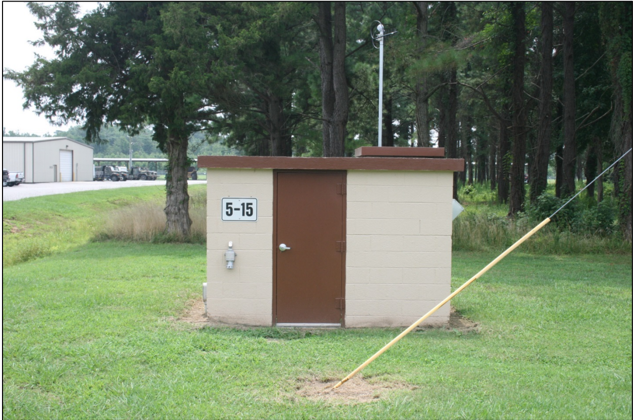
Figure 97: Building 5-15, north elevation
