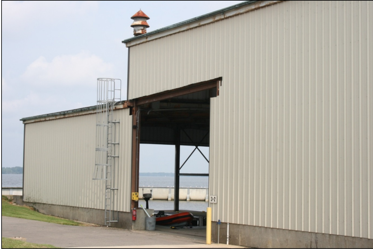
Figure 52: Building 3-2, exterior door detail, south elevation
